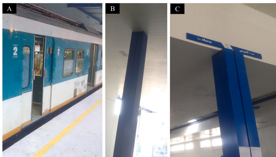
Fig. 3. Tunis train station – (A) train platform, (B and C) PVC coating at the station.
